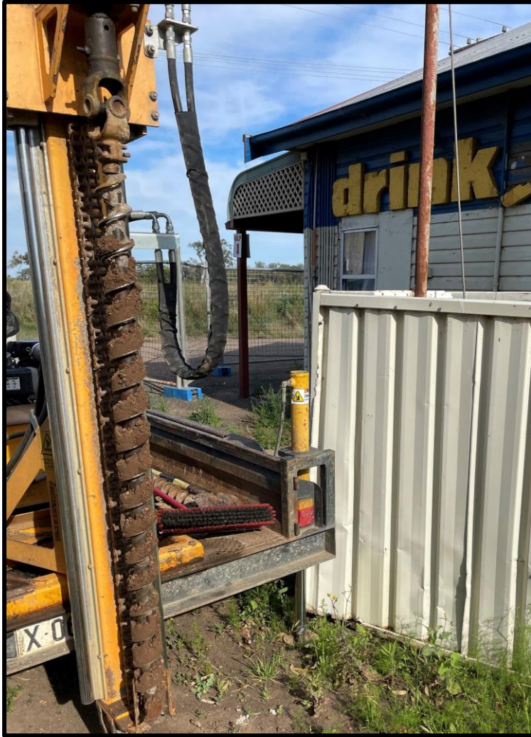
Figure 13. Drilling of S1. The fill layer consisted of a Dark Brown Medium Clay soil.
